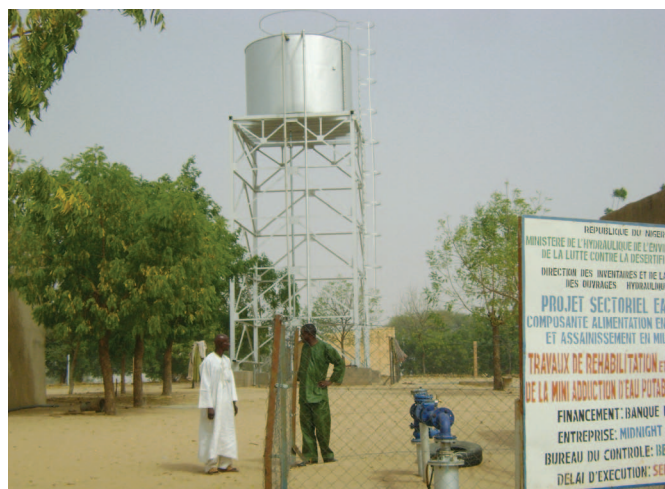
Overhead water tank for water supply system in Niger (Photo: Taibou Adamou Maiga)
