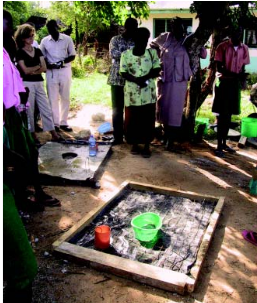
Fabrication of a concrete slab for a Fossa Alterna.
