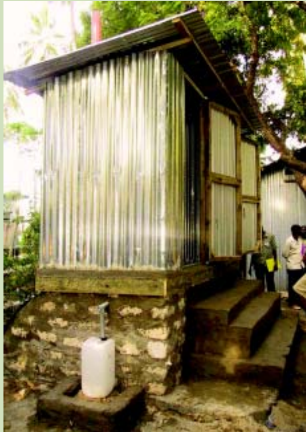
A urine diversion toilet near Mombasa where the jerrycan is used as a urine container.
