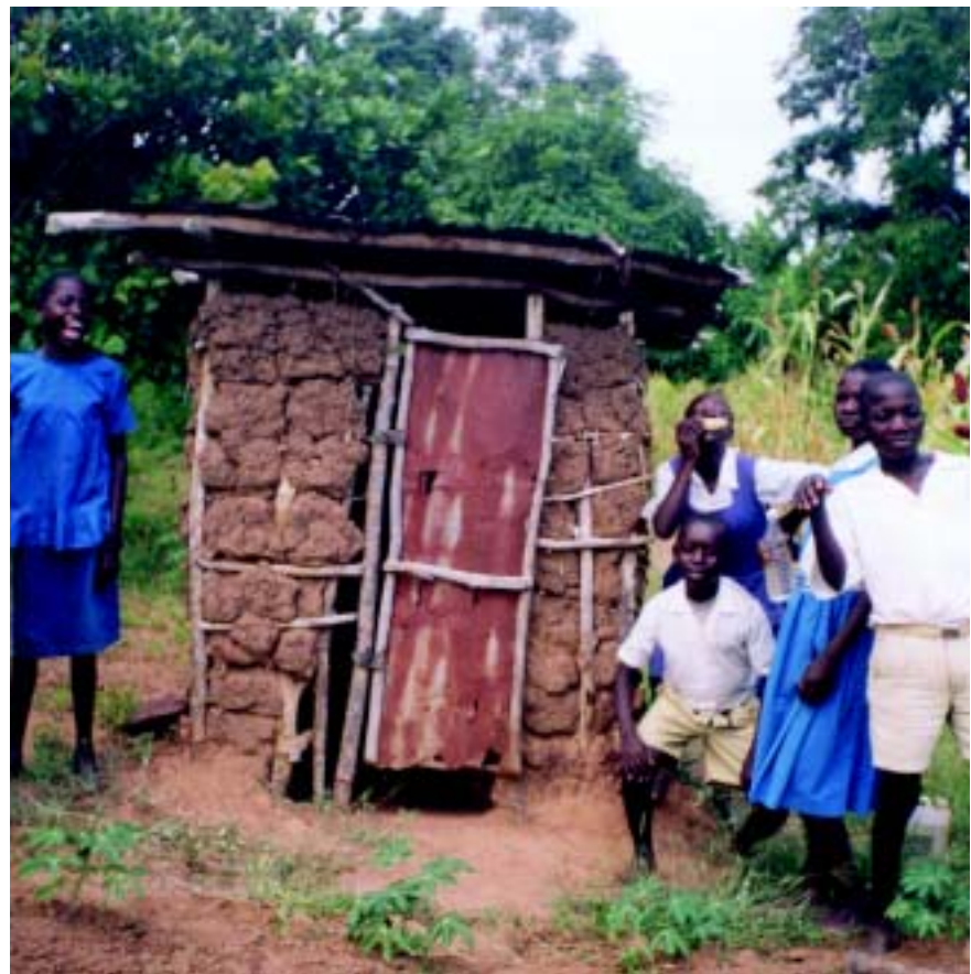
A poorly constructed pit latrine.
