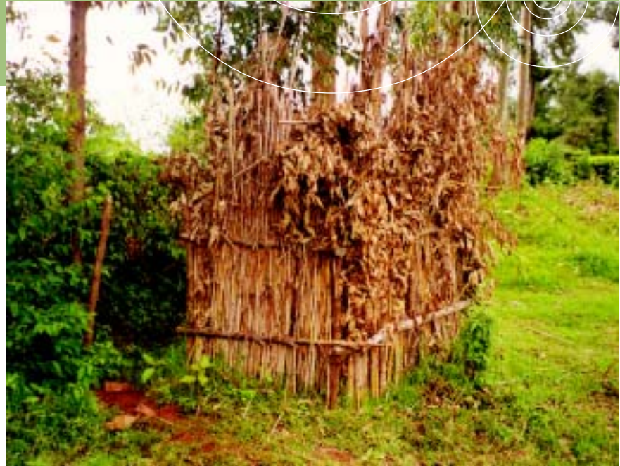
A simple pit latrine built using locally available materials.
