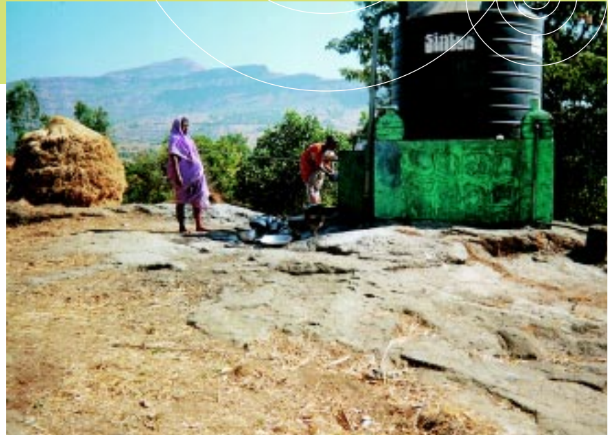
A storage tank and public standpost in Hadshi, Pune.
