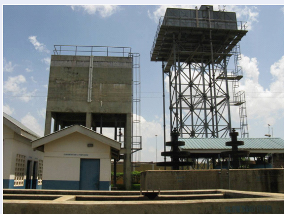
Ground and elevated water storage facilities. (Source: Hydroconseil)
