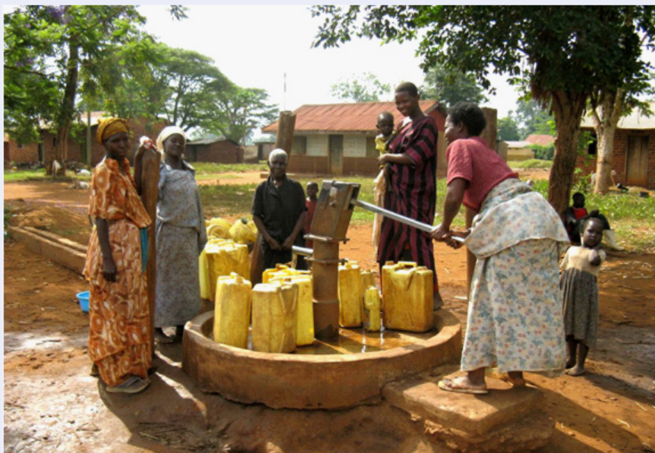
Women fetching water at a public water pipe (PWP). The PWP is installed over a borehole and households pay nominal fees to fetch water from this source. (Source: Hydroconseil)
