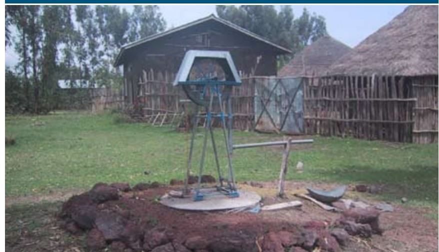
Figure 5. Sealed family well with new rope pump, Oromia Region
