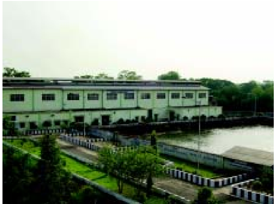
New River Pump House.
