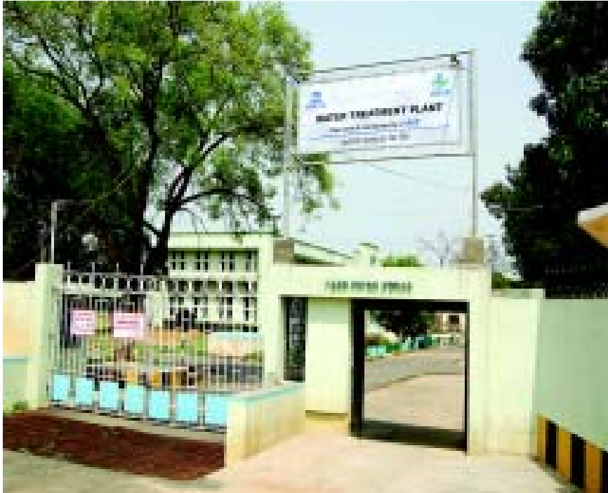
JUSCO's water works.
