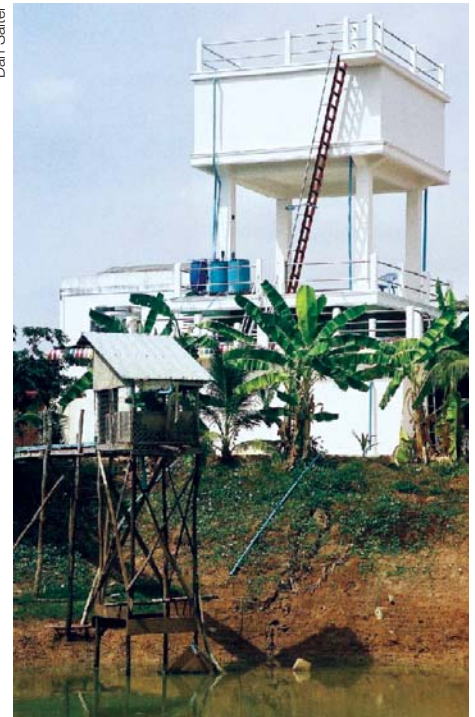
Piped water source and water tower in Cambodia
